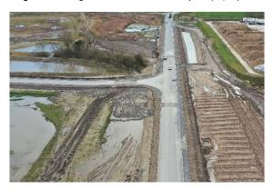
**Image 04:** Showing Topsoil works complete ready to receive seed
