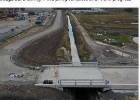
Image 03: Showing WCD Bridge preparation for Waterproofing
